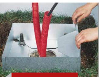
Reserves the space around the base of a lamppost, which will only be installed once the pavement is finished.
